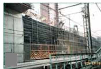
(b) wall under construction
