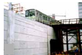
(c) completed wall
