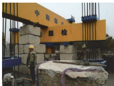
Fig. 5 Load test of the top-down loading
