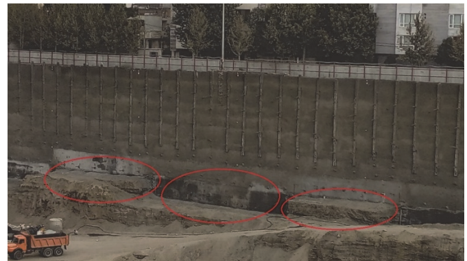
Fig. 4 Alternate-span excavation of 15 m length and 2 m thickness
