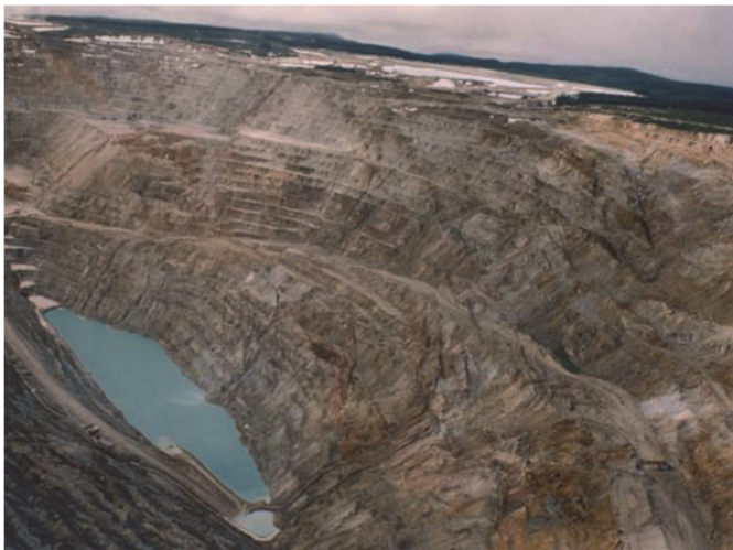
Fig. 12 Southeast wall: large-scale toppling failure (Brox and Newcomen 2003)
